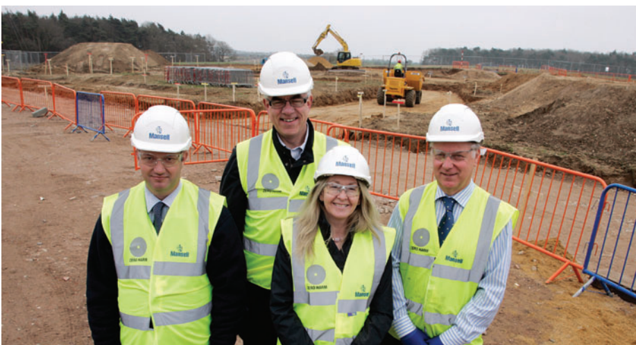
Mansell Senior Project Manager Neil Smith (left) and Site Manager David Rydlewski (right) on site with Scira's Einar's Strømsvåg and Anita Holgersen.
